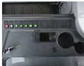
Centralized instrument switch panel
