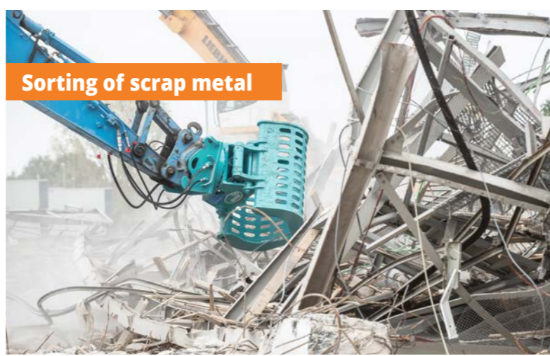
Separation of various construction materials
