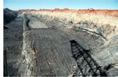
Overburden removal, bench, road & ramp levelling
