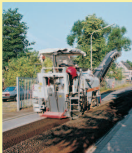
Another possibility: the RAP can also remain on the milled surface.
