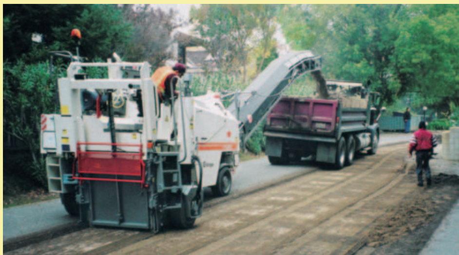
Little noise in spite of the powerful engine: soundproofing is a standard feature of the W 1000 F/W 1200 F, so that they can even be used without difficulty in residential areas.
